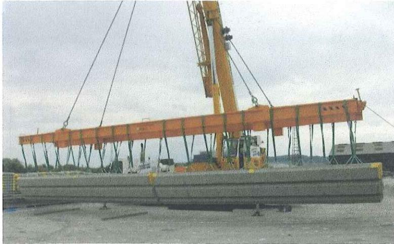
However, standard concrete mattresses are not permanent fixtures and they may be hooked and dragged out of position by trawl / anchor gear, exposing the cable. They act as 'sacrificial' protection in this case. The edges of the standard concrete mattresses may also induce localised scouring of the seafloor in strong current conditions.
